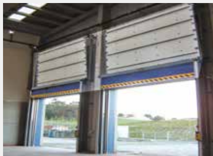
Speed door combined with sectional door.
