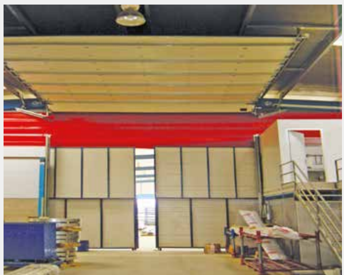
Speed door combined with sectional door.
