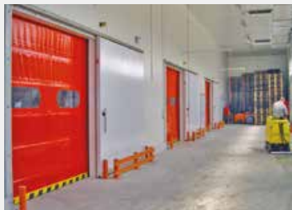
Speed door combined with sliding door.
