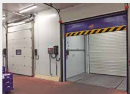
Speed door with sectional door and roller shutter door.
