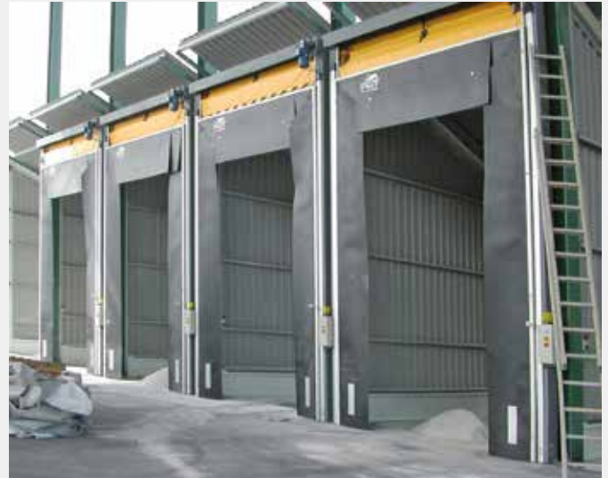
Speed door in silos combined with AF shelter.
