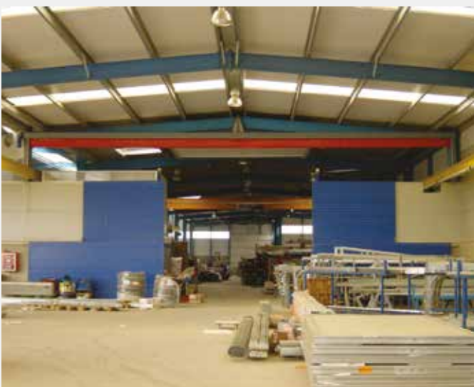
Speed door with bridge crane.
