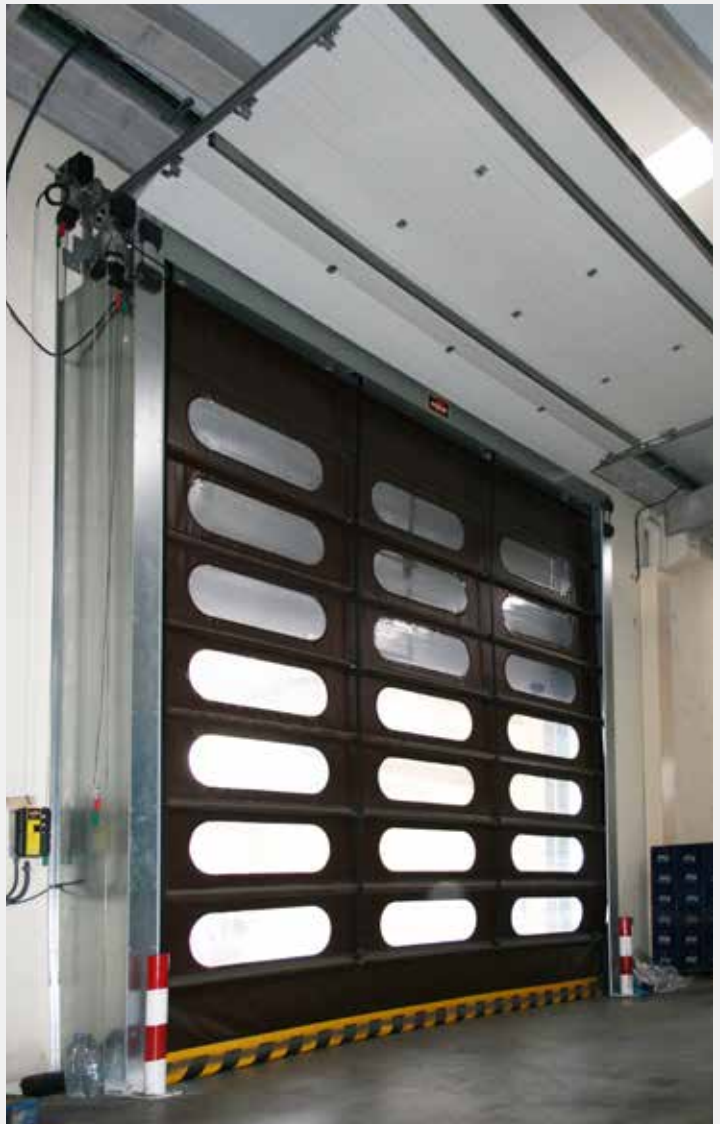
Speed door combined with sectional door con union closure.
