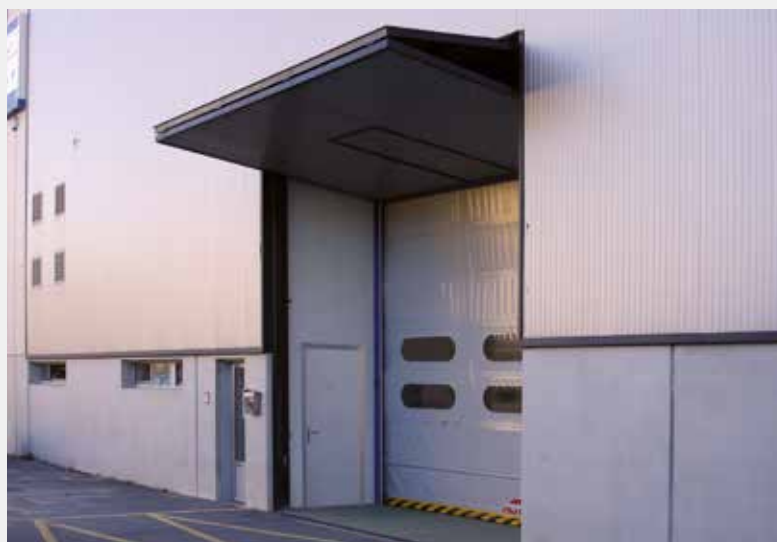
Speed door with lateral closure and pedestrian door.
