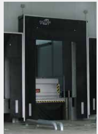
Lifting table installed inside with aluminium loading bridge.
