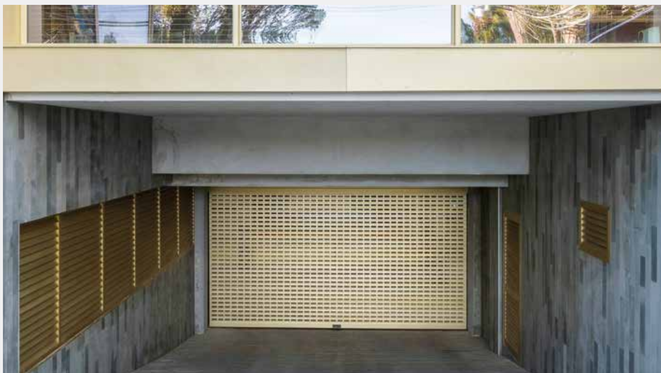
Door Alumir C80T with gold anodized finishing without polycarbonate for greater ventilation.
