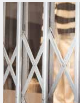
Detail of the steel scissor door.
