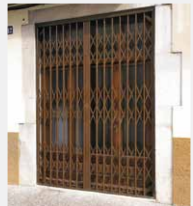
Detail of the steel scissor door.
