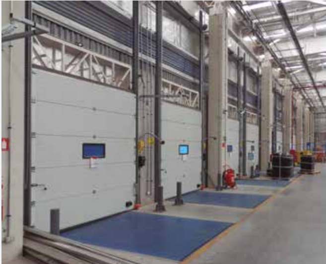
Sectional doors, Hydra dock levellers and Versalight led lighting in loading bay.
