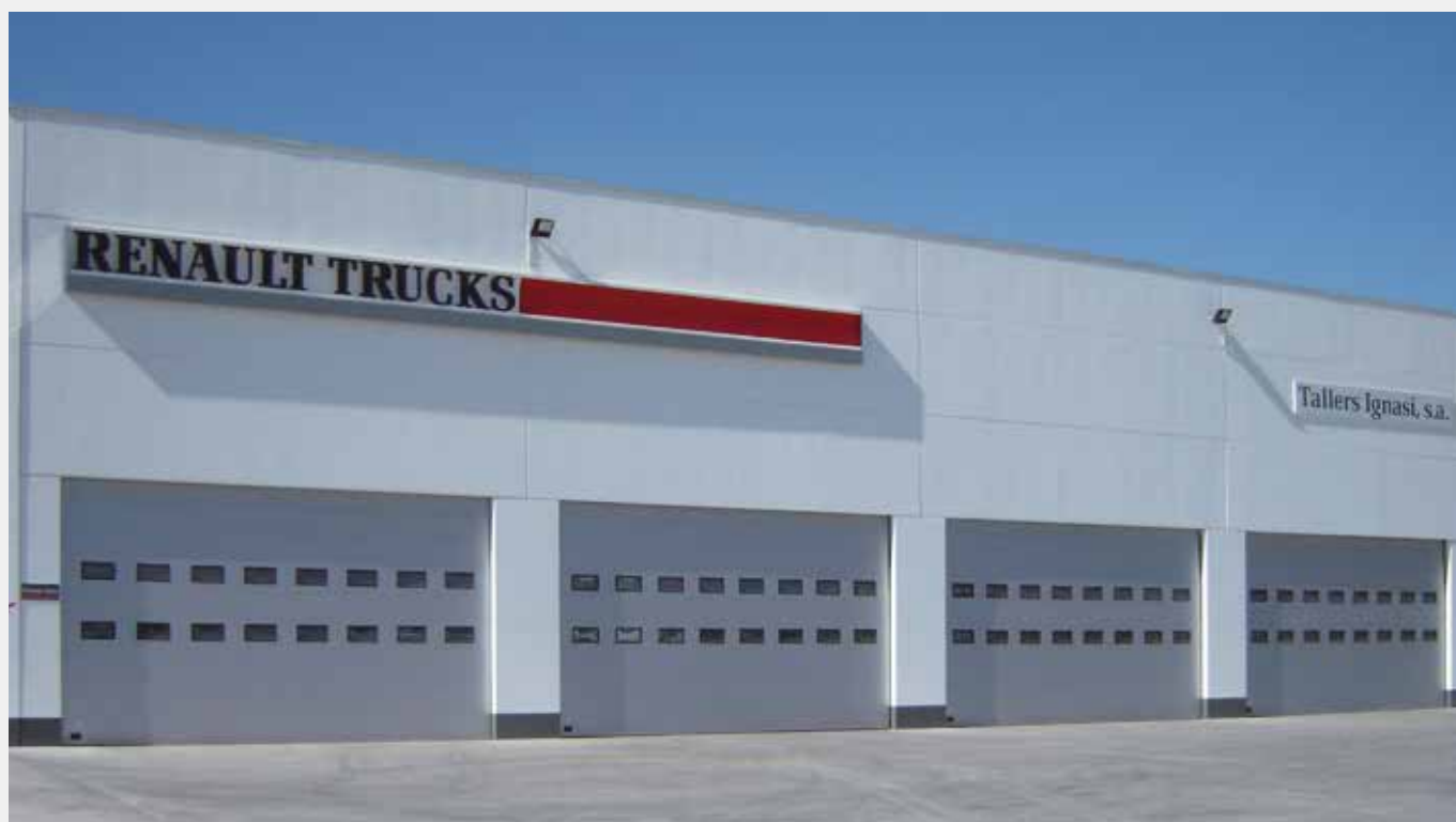
Sandwich panel sectional doors with peepholes in car dealer.
