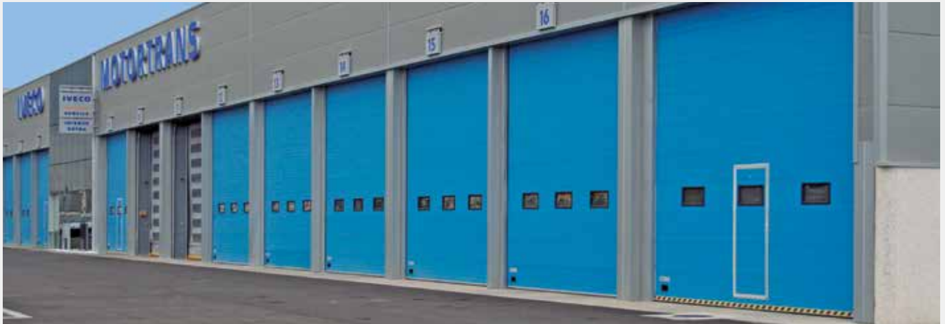
Sandwich panel sectional doors with peepholes and pedestrian door in car dealer.
