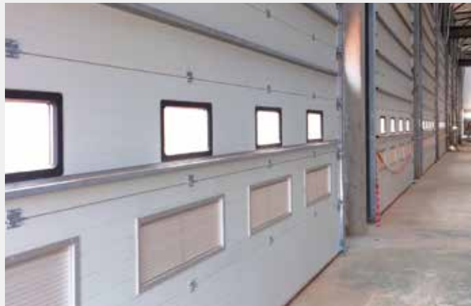
Interior view of door with rectangular peephole and ventilation grille. Peephole 610 x 350 mm. Grille 1050 x 360 x 35 mm.
