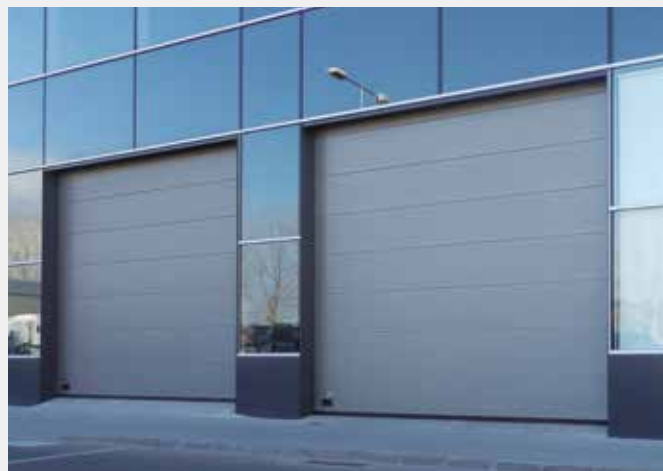
Micro-profiled sandwich panel sectional door in automotive company.
