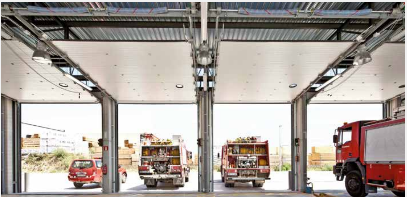
Interior view of sandwich sectional doors in fire station.
