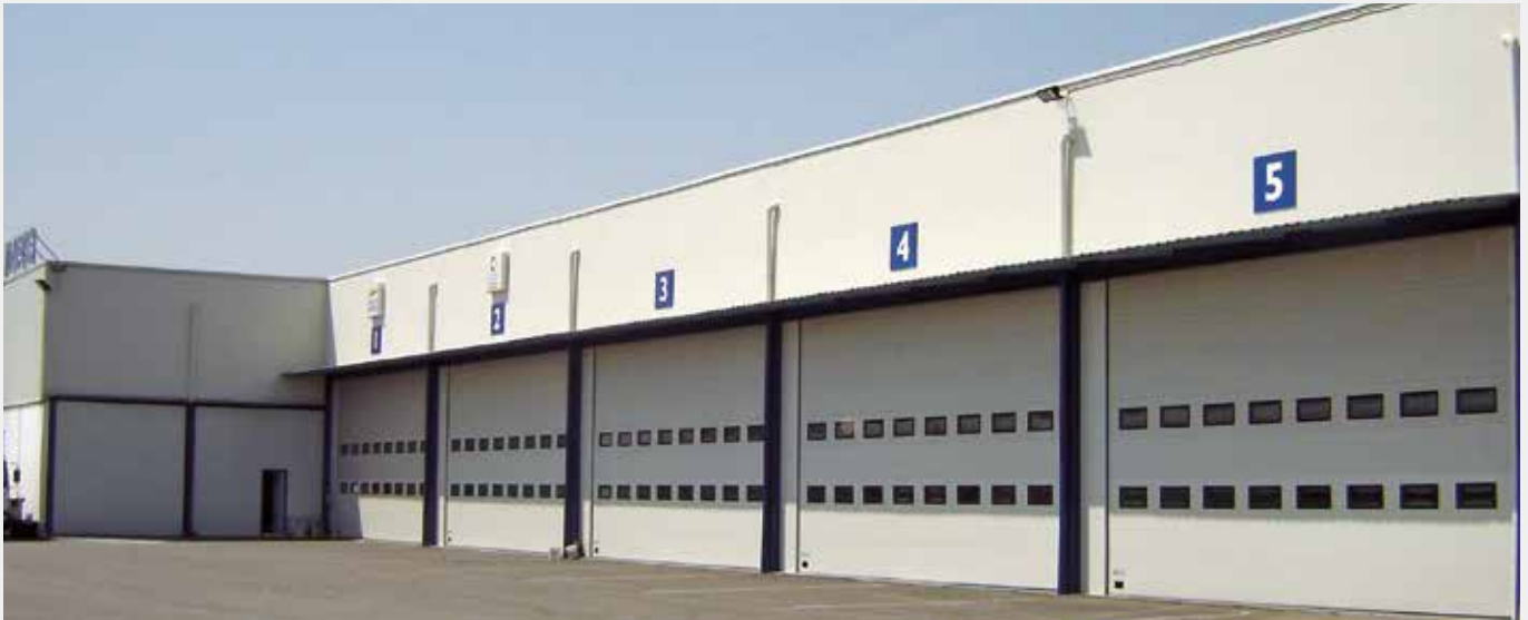
Sandwich panel sectional doors with peepholes.
