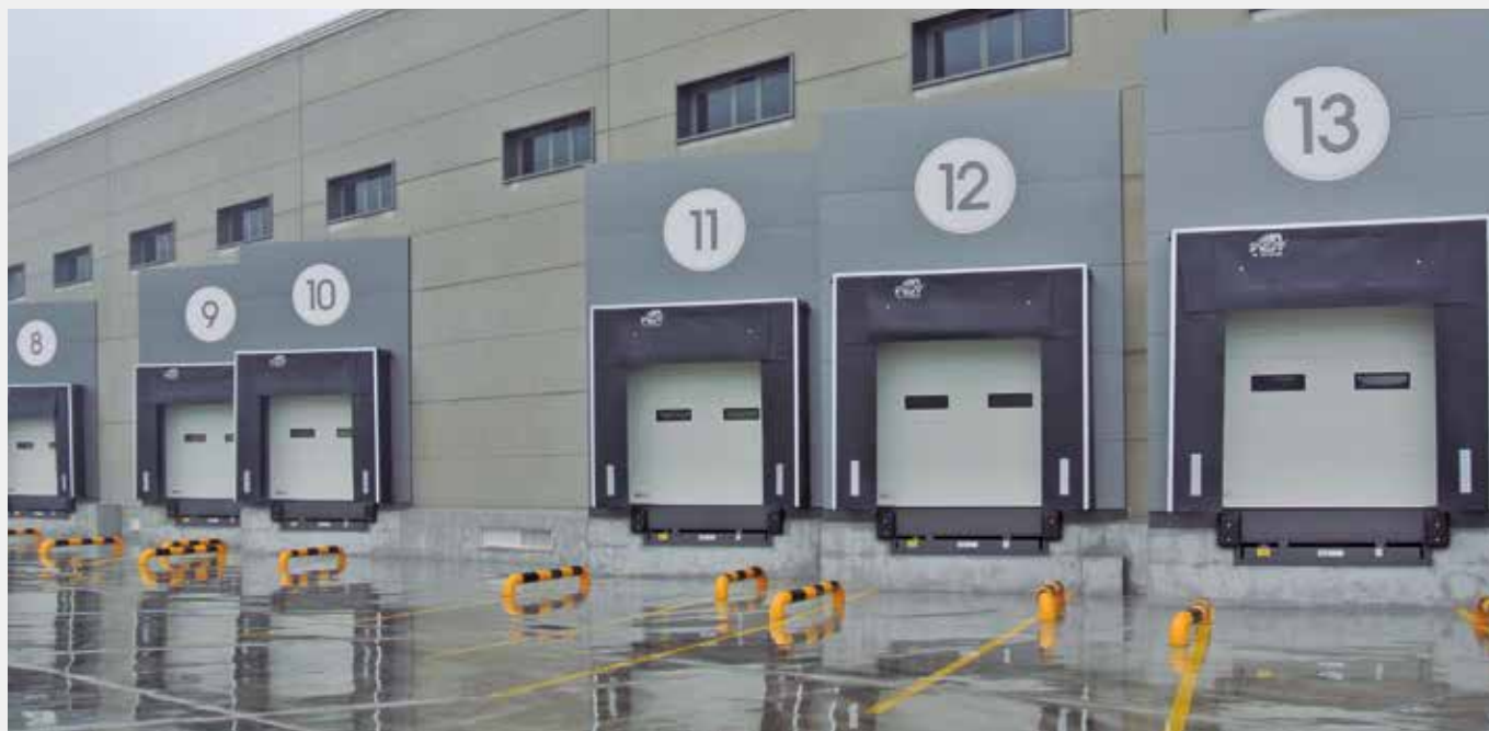
Sectional doors with peepholes in loading docks.
